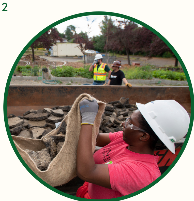
2 Volunteers removed over 50,000 SF of pavement freeing the soil below and preparing the land for garden beds
